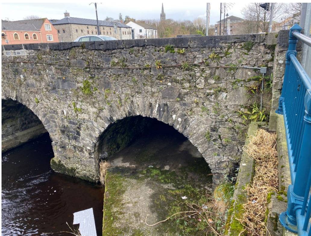
Plate 8 Downstream elevation of Arch 7, showing the concrete platform across its base and extending southwest, and the southwest abutment. Taken from southwest.
