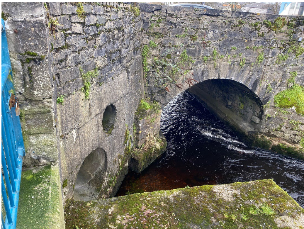
Plate 7 Upstream elevation of Arch 7, covered by angled concrete culverts with Pier 6, partially covered, and Arch 6. Taken from the southeast.
