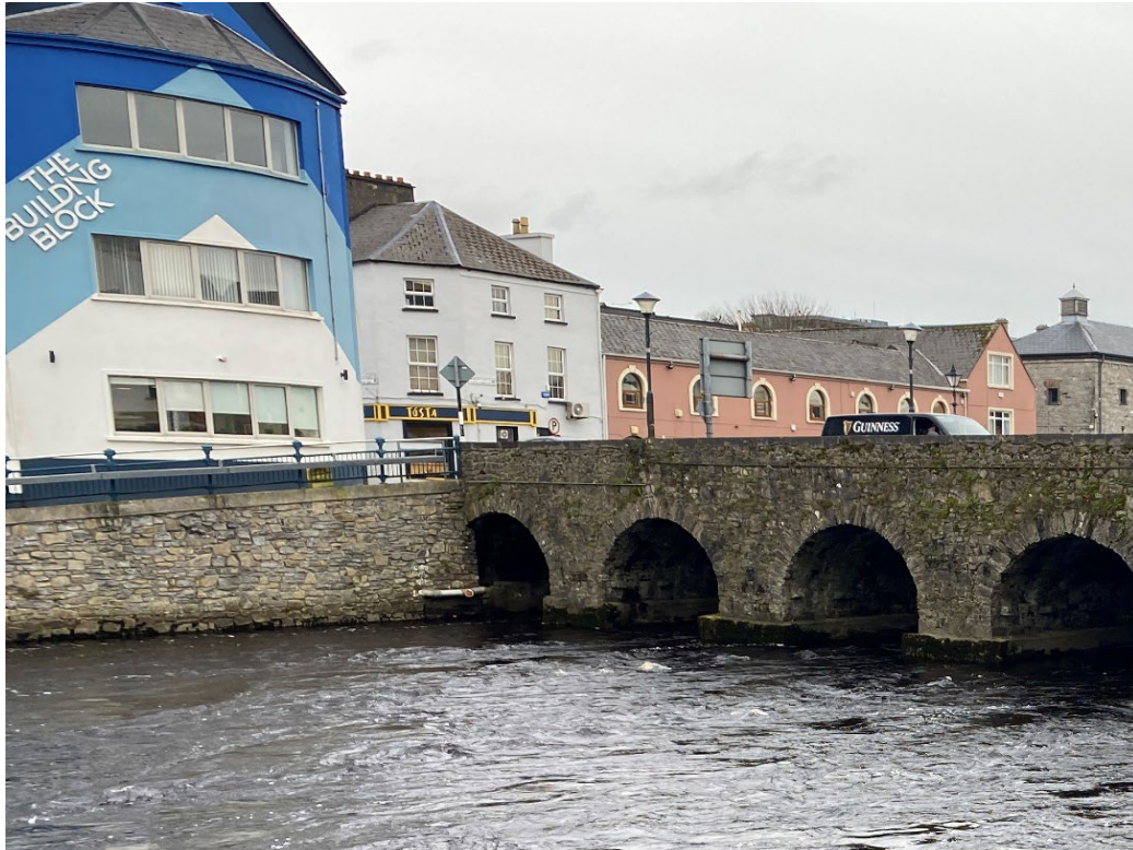
Plate 6 North-western abutment, showing modern stone quay wall encroaching on downstream opening of Arch 1, and pipe exiting Arch 1. Taken from the southwest.
