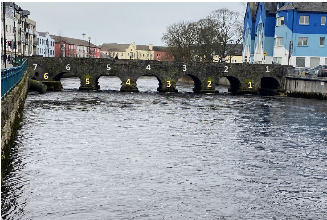
Plate 3 Upstream elevation of Markievicz Bridge, taken from the southeast. Arches labelled in grey and piers labelled in yellow.
