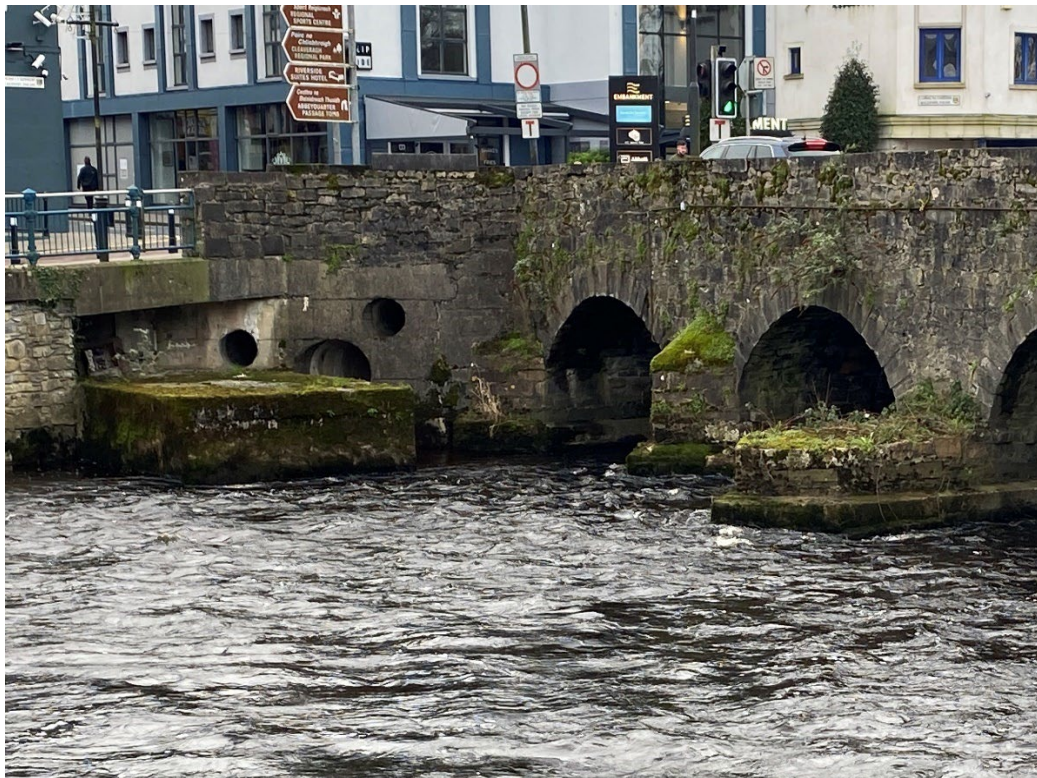
Plate 11 Upstream elevation showing where Arch 7 has been covered by a modern, angled abutment with concrete culverts. Pier 4, with trapezoidal cutwater, is visible to the right. Taken from the northeast.
