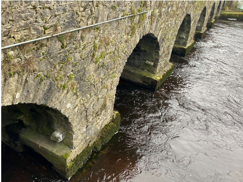
Plate 10 Downstream elevation showing difference in voussoir decoration. Taken from the northwest.
