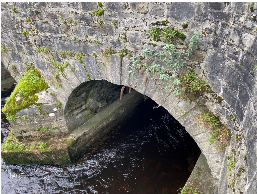
Plate 9 Upstream elevation showing Arch 1, with voussoir and cutwater details. Evidence of centering visible along the pier wall. Taken from the northeast.
