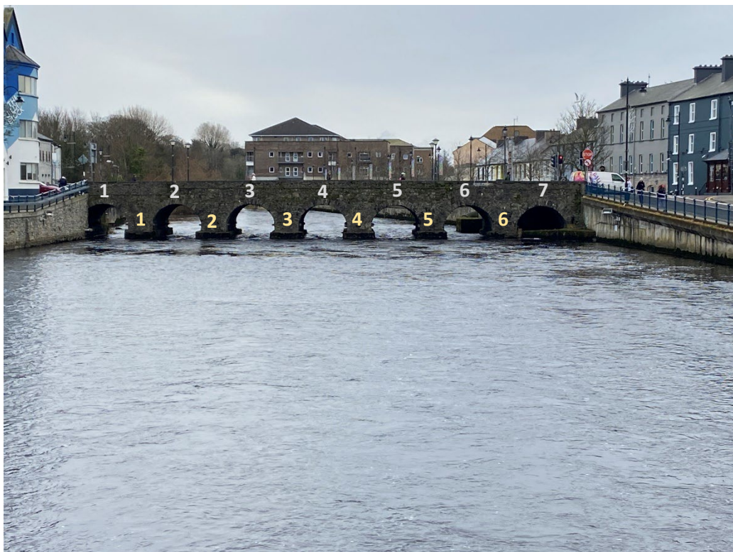
Plate 4 Downstream elevation of Markievicz Bridge, taken from the west. Arches labelled in grey and piers labelled in yellow.
