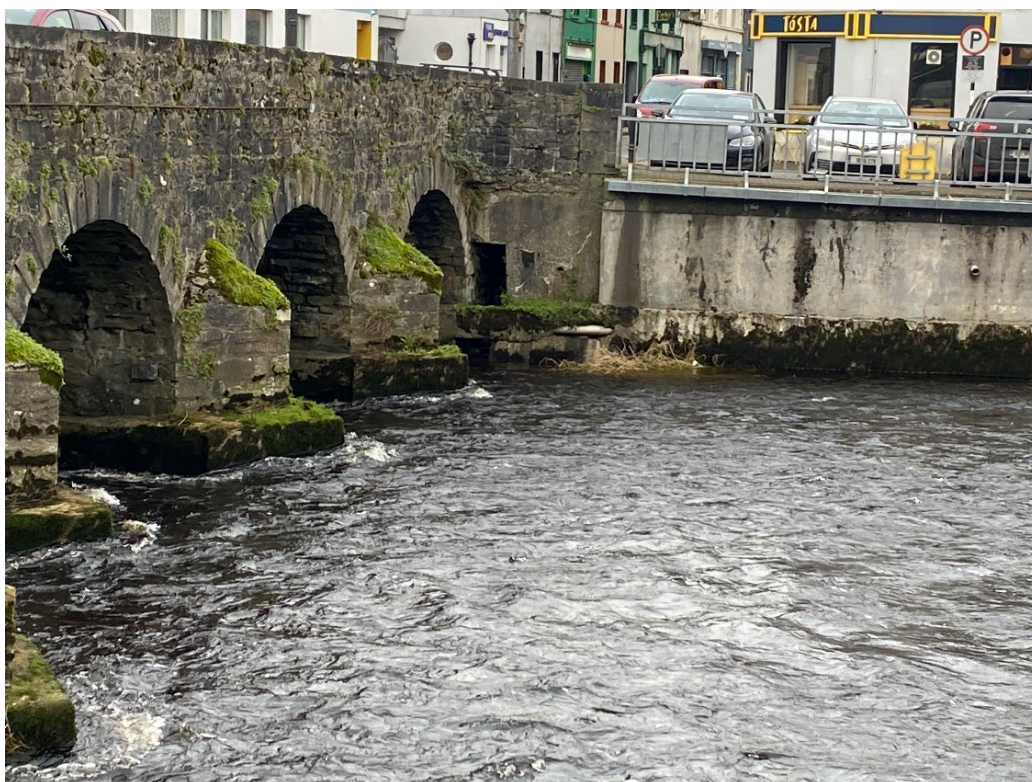
Plate 5 North-eastern abutment taken from the south. Note the opening perpendicular to Arch 1, crossed by a concrete-encased service.
